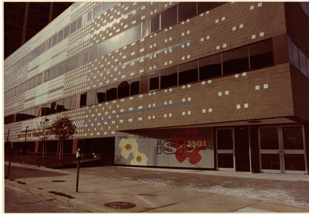
Fig. 6. ISI headquarters in the late 1970 at 3501 Market Street, Philadelphia, PA designed by Venturi Scott Brown Associates.
