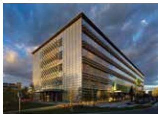
EEEL uses 78 per cent less energy compared to a conventional laboratory building. Photo by Tom Arban
